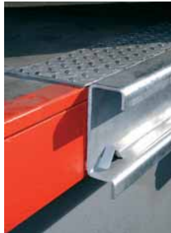
Galvanized steel plate fixed on top of dock with flush fixings.
